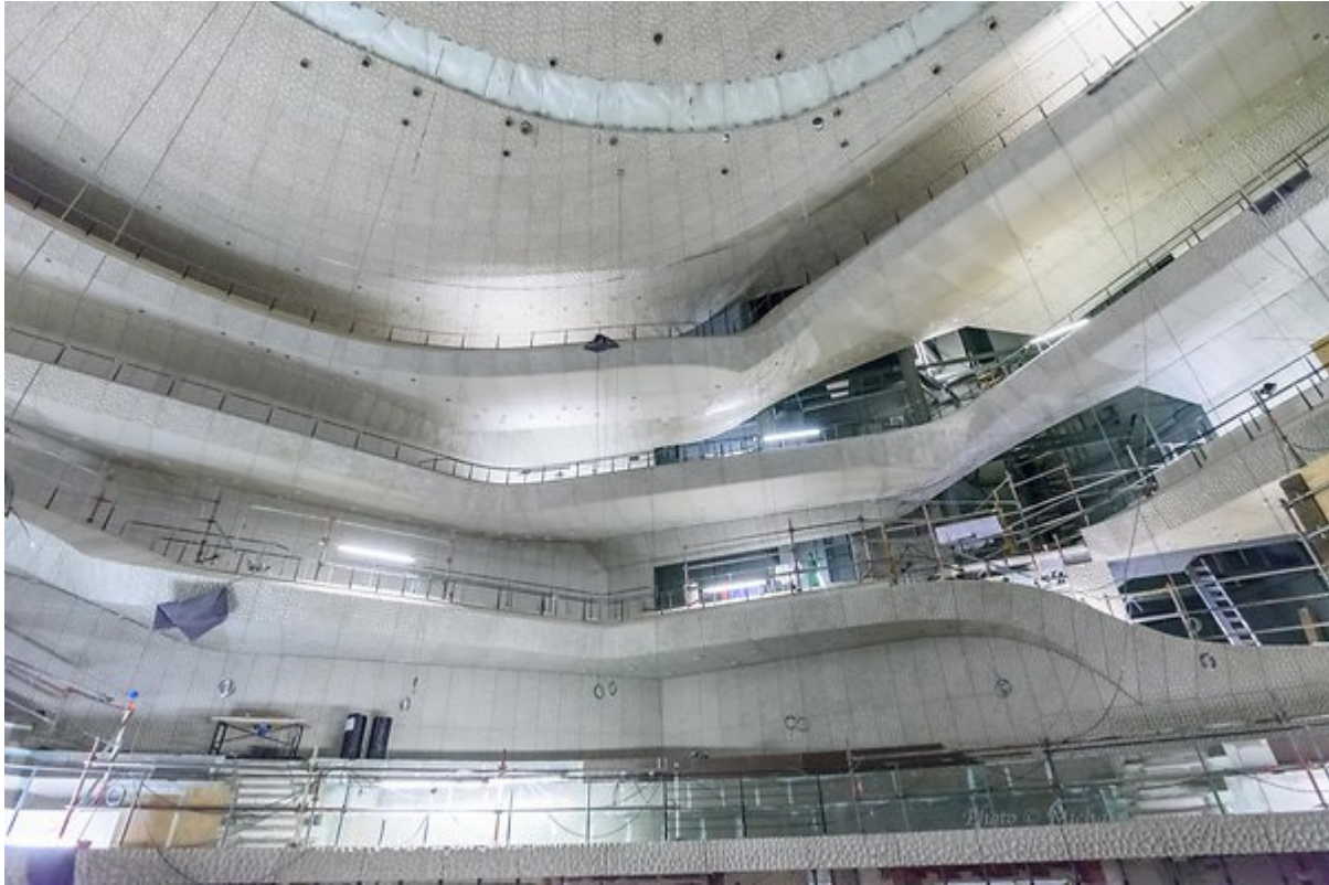
Grooves and hills scatter the sound: The “White Skin” of the Elbphilharmonie
