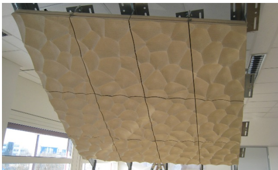
The 10,000 gypsum fiber panels, each having a unique structure for an optimal distribution of sound. © Peuckert
