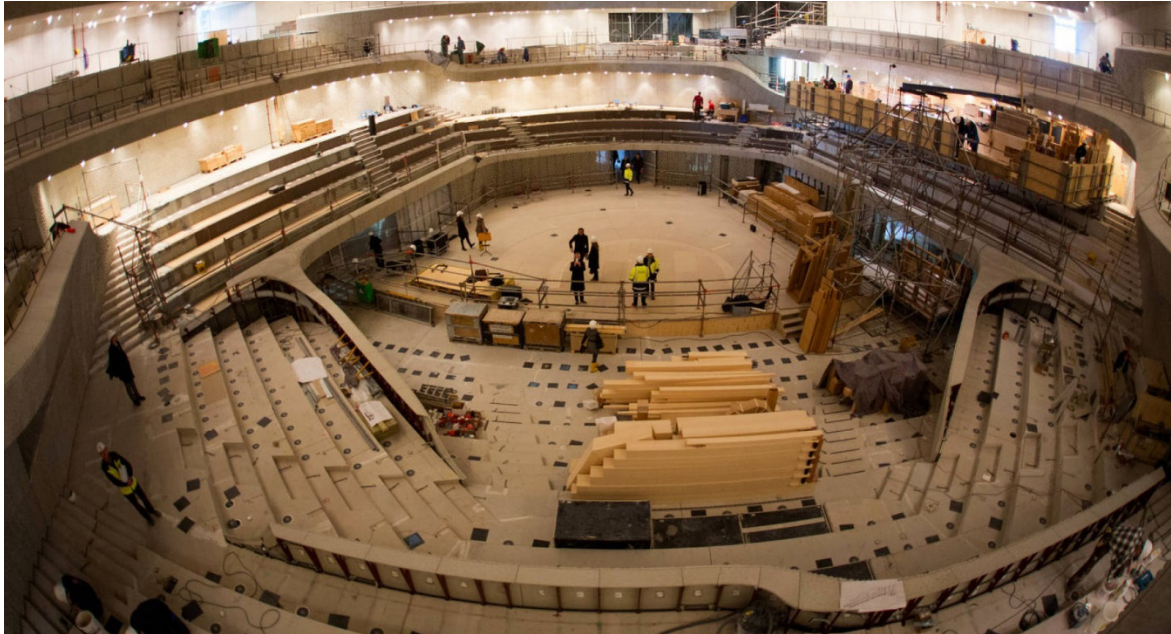
Construction work of the Great Concert hall in early February. A special wall covering, the so-called "white skin" is intended to ensure good acoustics. © dpa
