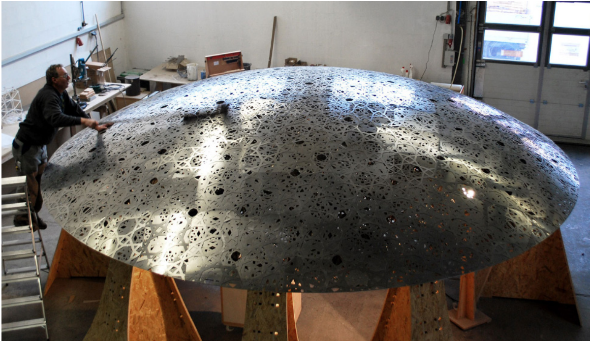
Louvre Abu Dhabi Prototype in fabrication (Image: One to One)
