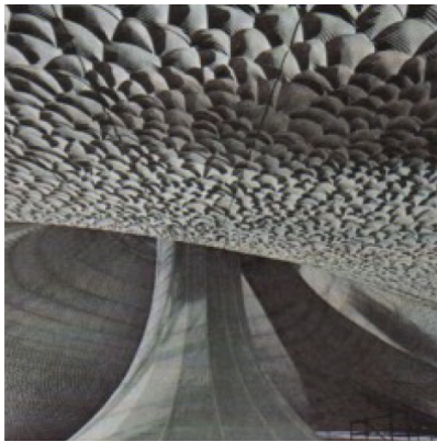
The white ceiling in the Great Hall. Chaos creates harmony - the surface must be irregular, such that the sound is scattered evenly, explains Koren.
