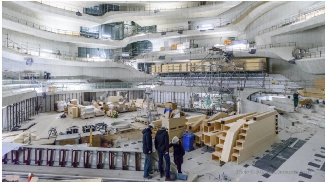
The construction of the great hall. A special wall cladding system, the so-called "white skin" will provide for good acoustics
