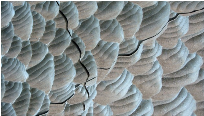
Elbphilharmonie: The so-called "White Skin" consists of 10,000 panels created on the computer
